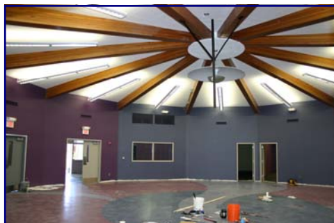
The interim performing arts building is nearing completion.
