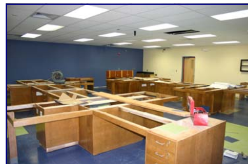
The new science co-lab is nearing completion.
