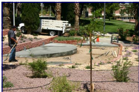
M&O is putting the finishing touches on the meditation garden.
